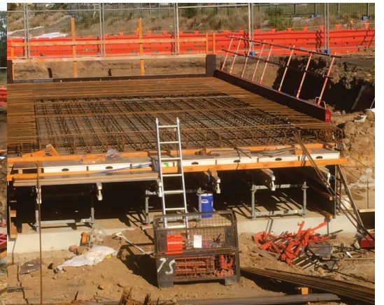
Ready for concrete
