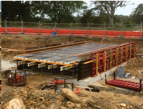
Suspended slab culvert works
