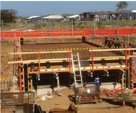
Reo placement on suspended slab
