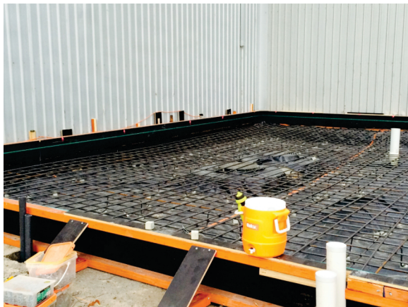
Wash-down slab prep
