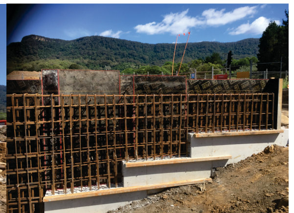
Retaining wall reo
