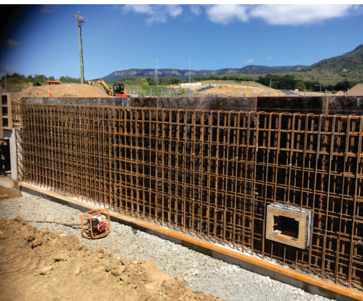
Reo for retaining wall
