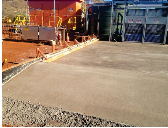
Brockman 4, Waste Water Services Containment slab for waste water treatment plant
