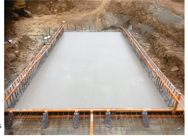
In situ Culvert works
