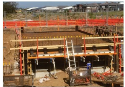
Reo placement on suspended slab
