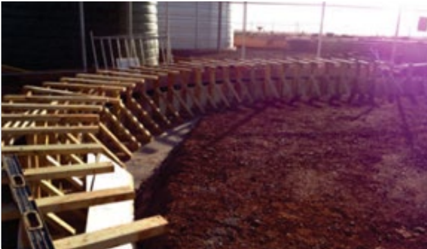
West Angelas, Waste Water Services Ring beam for waste water treatment tank
