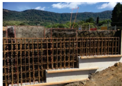
Retaining wall reo
