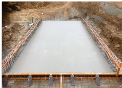
Insitu Culvert works
