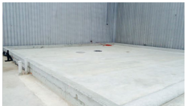
Wash-down slab completed
