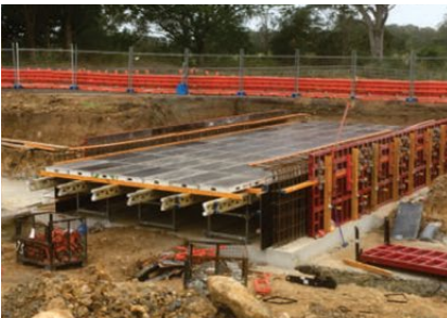
Suspended slab culvert works
