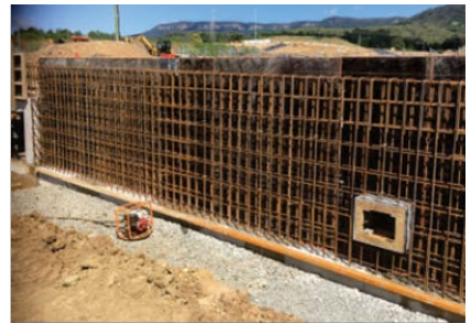
Reo for retaining wall
